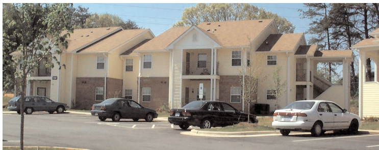
Partnership Village is a special needs development that provides supportive services for formerly homeless individuals and families.
