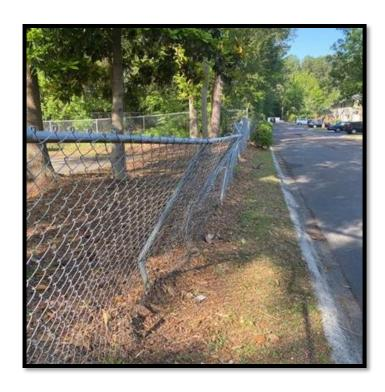
DEFICIENCY 3 - Outside: FENCE DEMONSTRATES SIGNS OF COLLAPSE.
