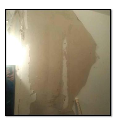
DEFICIENCY 1: Interior wall has a hole of any size that penetrates to the adjoining room or space.
