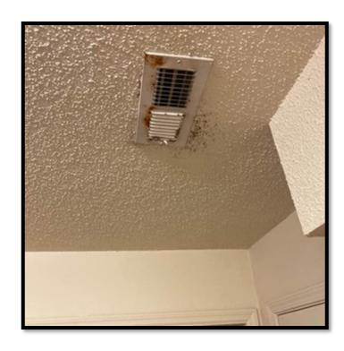
DEFICIENCY I — UNIT: PRESENCE OF MOLD-LIKE SUBSTANCE AT VERY LOW LEVELS IS OBSERVED VISUALLY.
