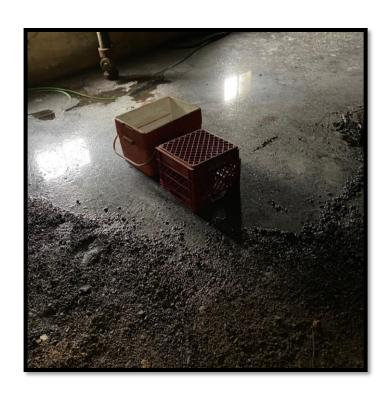
Deficiency 4 — Inside: FOUNDATION IS INFILTRATED BY WATER.
