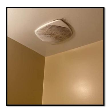
Deficiency I - Inside: Presence of mold-like substance at very low levels is observed visually.
