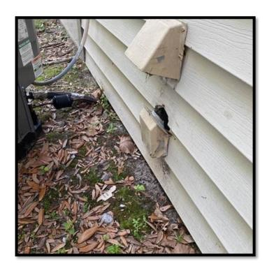
Deficiency 4 - Outside: Exterior dryer vent cover, cap, or a component thereof is missing.
