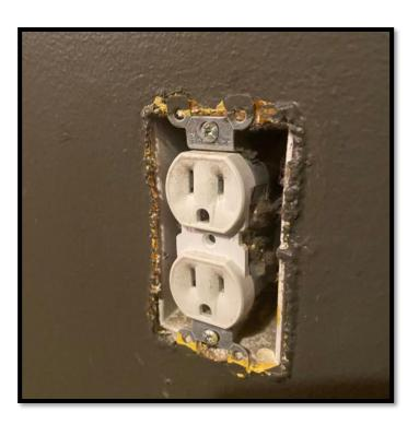
DEFICIENCY I — UNIT: EXPOSED ELECTRICAL CONDUCTOR.
