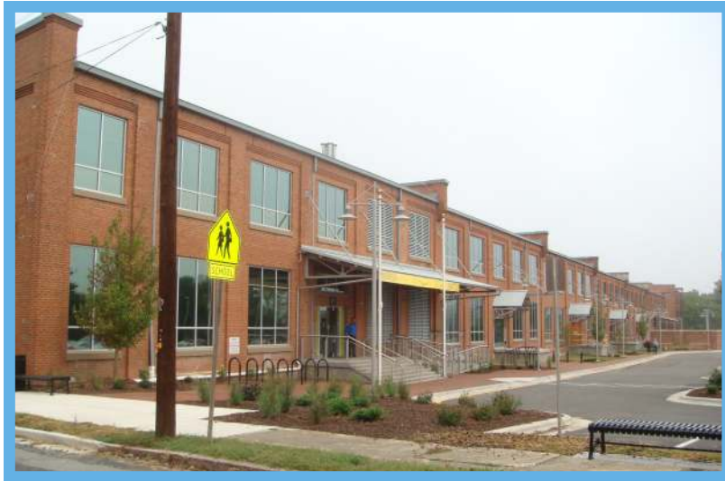
A former Liggett & Myers tobacco warehouse in Durham, NC, the Carmichael Building, is now home to lab, research, and office space for Duke University's Molecular Physiology Institute. New Markets Tax Credits helped make this rehabilitation possible.
